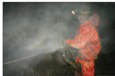
Drilling and ready to blast! J. Fisher and R. Brandstetter photos.
