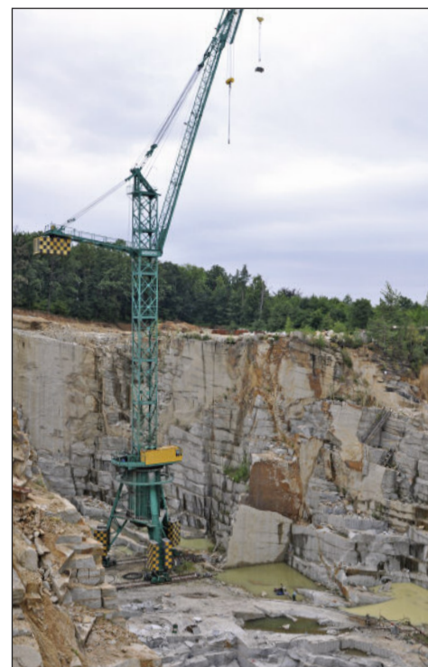
Wekom II Quarry with giant crane used for transport of granite blocks and machinery. T. Praszkiar photo.
